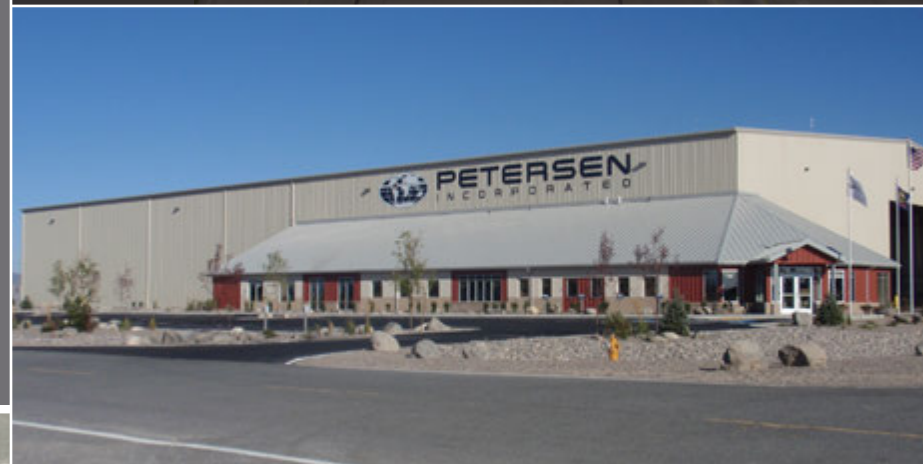
Idaho Facility, Pocatello, ID
